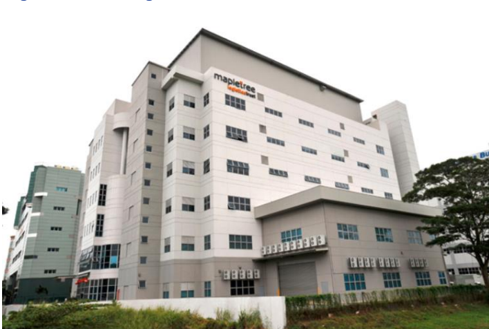
Figure 7: 7 Tai Seng Drive before asset enhancement
