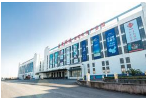
Figure 20: Fu Heng Warehouse
